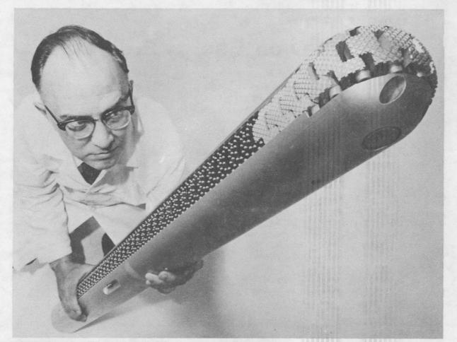
MODEL OF EXPERIMENTAL continuous chain bit, held by Dick Ashmore (ret.), shows cutting surface located on face of the chain, which advanced to bring new cutting surface into position. Despite promising initial test results, advanced development and testing were dropped.
